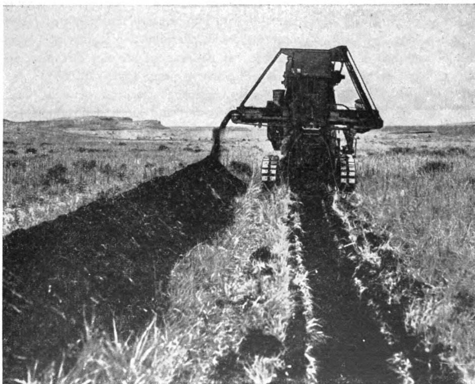
Figure 56. Ditcher digging trench for tile drain.
